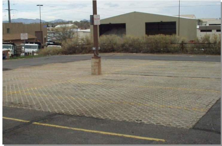
Photograph CGP-1. Concrete grid pavement installation in a parking area. The concrete segments along the perimeter of this installation showed wear that could have been mitigated with a concrete perimeter barrier.
