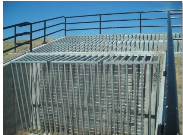
Photograph OS-5. Interruptions in the horizontal members of this trash rack and the spacing of the vertical members allow easier access to clean the water quality grate. A raking tool can be used to scrape the water quality trash rack.
