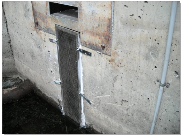
Photograph OS-3. Trash rack after repair.
