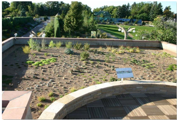
Photograph GR-5. A continuous green roof system at the Denver Botanic Gardens. It is a predominantly extensive system with some intensive areas. Photo courtesy of Denver Botanic Gardens
