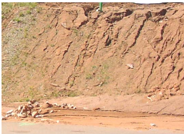
Photograph 7-2. Erosion is a common occurrence during construction activities, which can result in sediment movement off site and deposition in waterways when not properly managed. (Photo courtesy of Douglas County)
