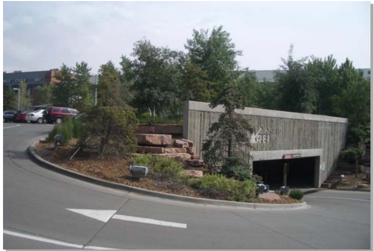
Photograph GR-6. Intensive green roof installation above a parking garage.
