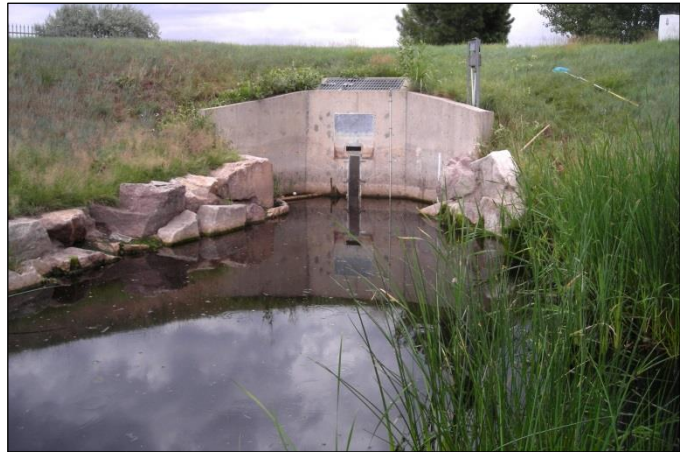
Figure 5.7-4. Micropool and Outlet Structure
