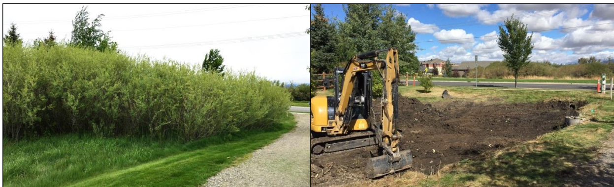
Figure 5.7-6. Detention Basin Deferred Maintenance
