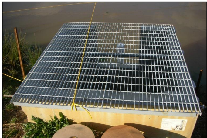
Figure 5.8-5. Outlet Structure Trash Rack
