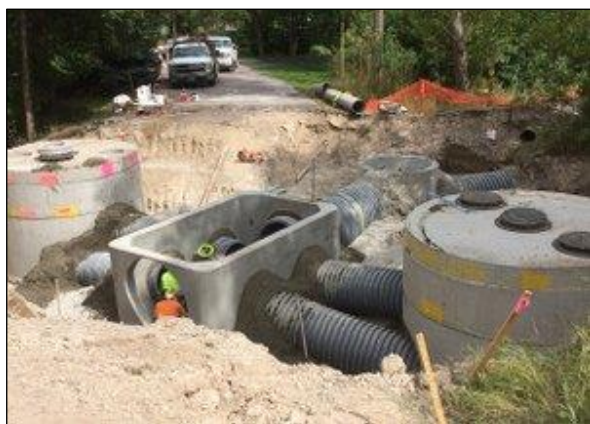
Figure 5.9-1. Proprietary Treatment Device Installation
