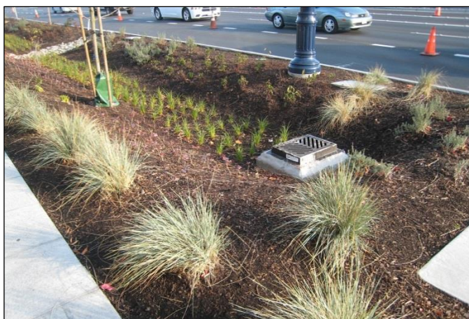
Figure 5.3-5. Online Bioretention Area with Overflow Outlet Structure
