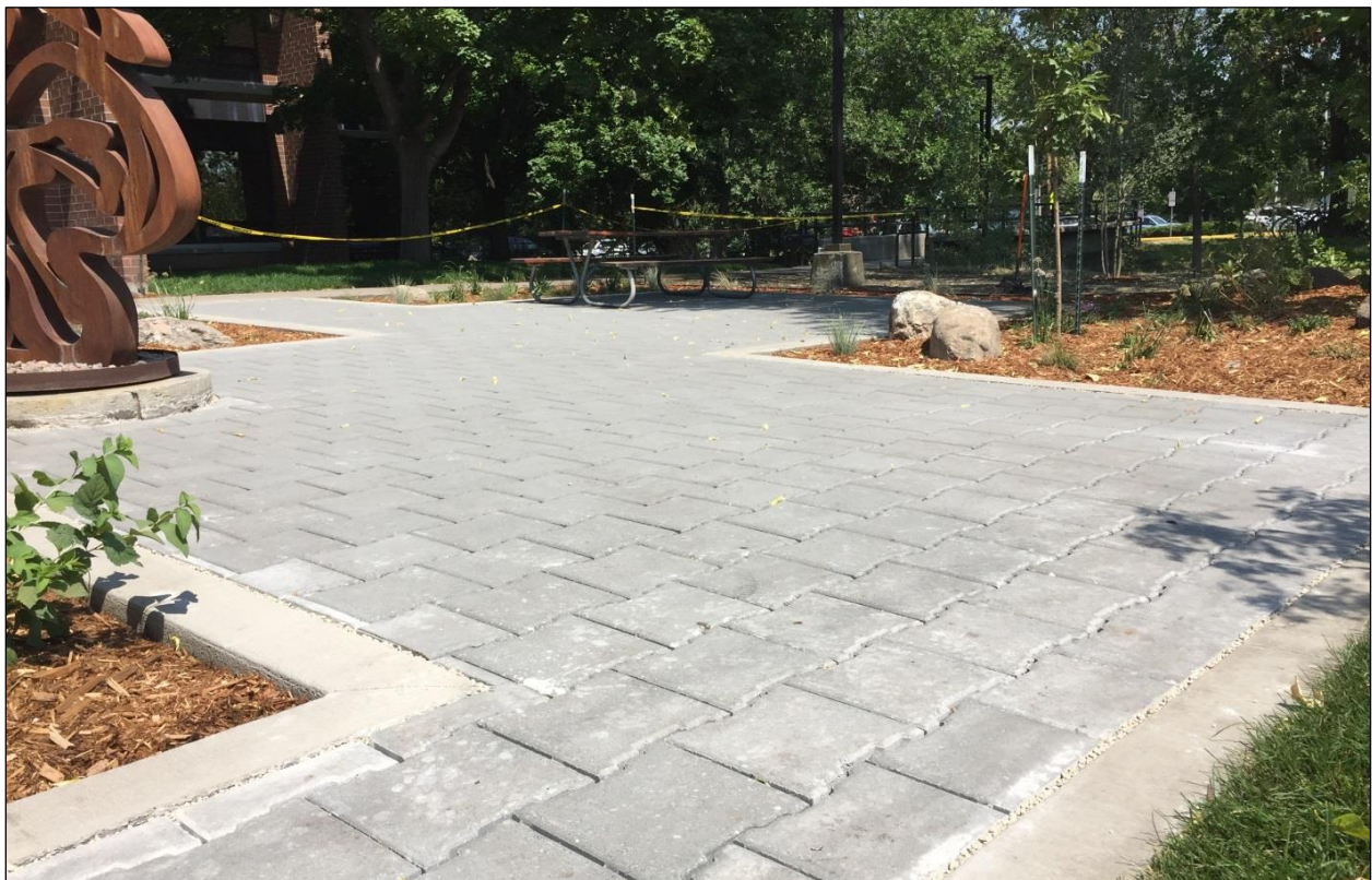
Figure 2-5. Permeable Interlocking Concrete Pavers Walkway Application
