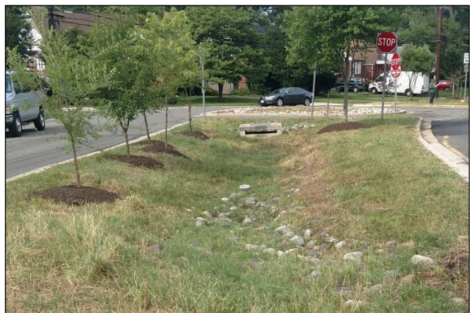
Figure 5.2-2. Infiltration Basin with Outlet Structure Source: HDR
