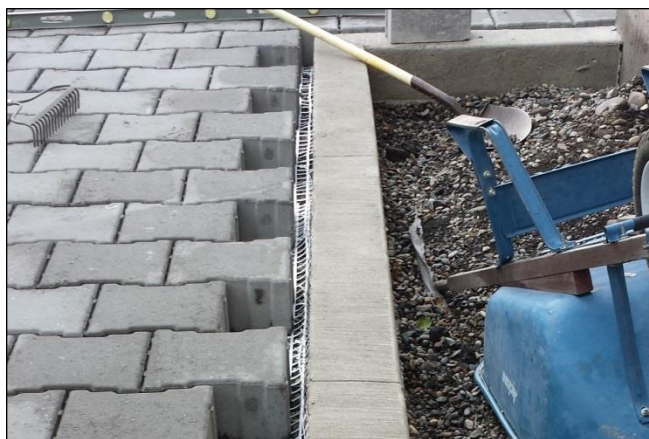
Figure 5.4-7. PICP Installation
