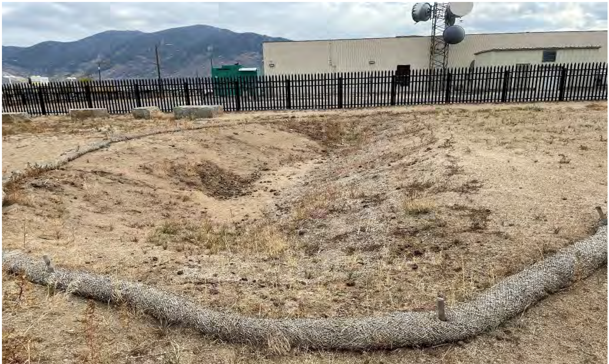
Photo 4 – Example of Pond needing revegetation and lack of stabilization
