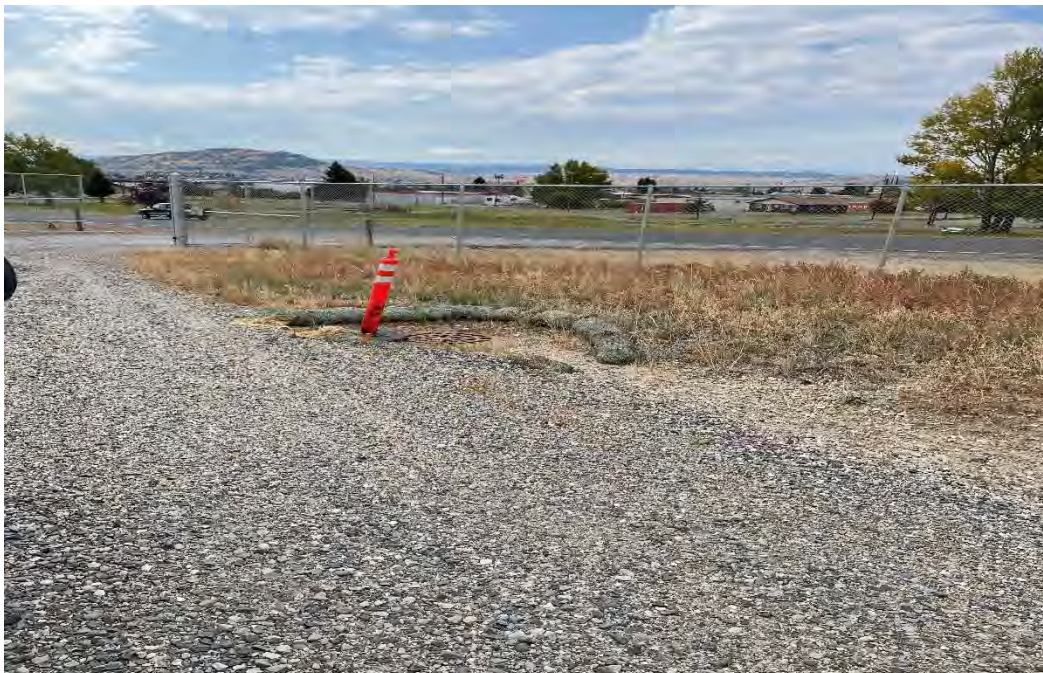
Photo 2 – Replace straw waddle with rock waddle or rock check dam to protect inlet
