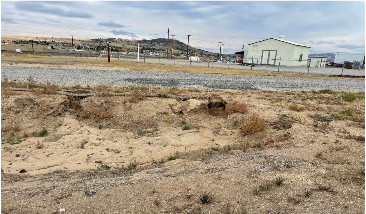
Photo 4 – Example of Pond needing revegetation and lack of stabilization
